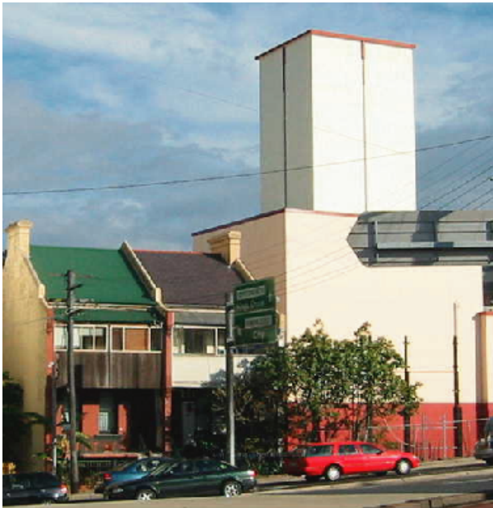
Emission stack nestled near Sydney homes
